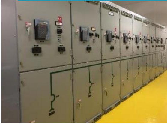
MV Switchgear Lineup
