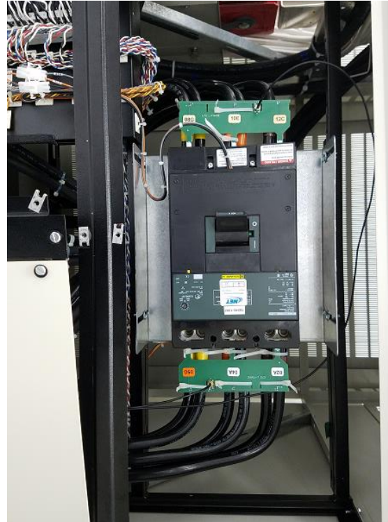
Molded Case Breaker Cables
