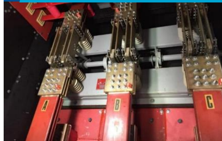
Generator Circuit Breakers
