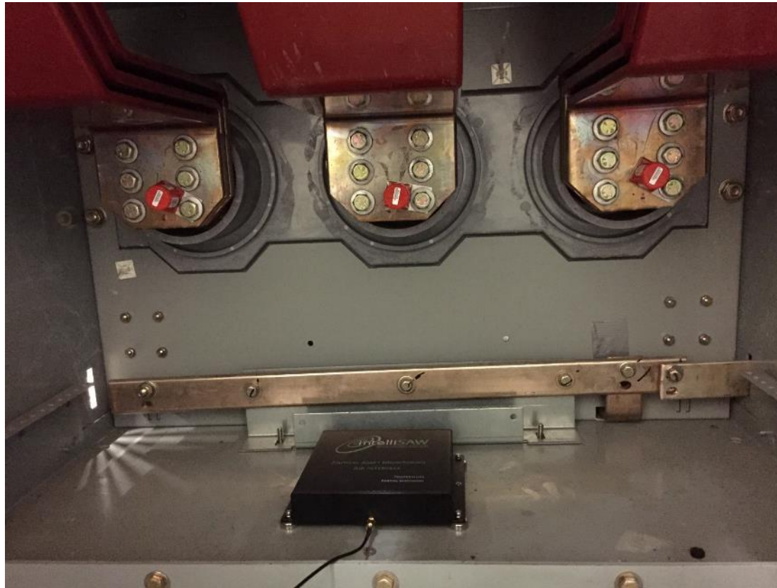
PD and Temperature Monitoring
