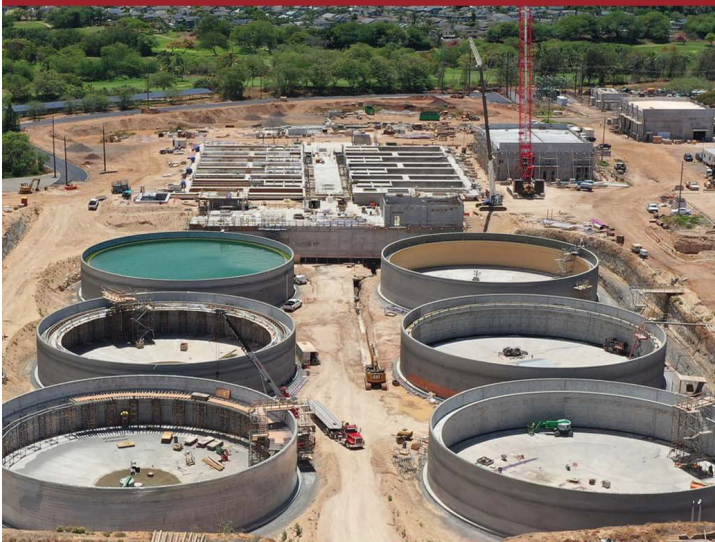
Tank Project: 6 x 2.0 MG Clarifiers — Honolulu WWTP
