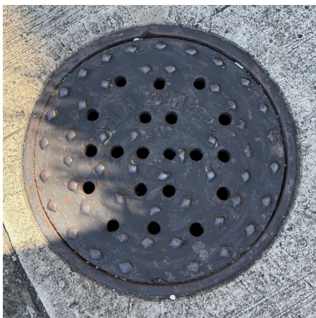
An original manhole cover on the sidewalk fronting the historic building. The cast lettering of "HB&M Co." stands for The Honolulu Brewery & Malting Company.
