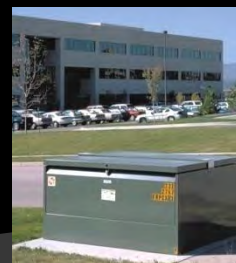
Pad Mounted Switches
